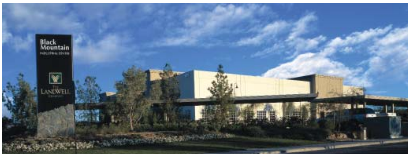
Black Mountain Industrial Center is one of several industrial complexes in the Henderson area.
